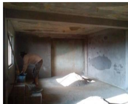
Figure 33: Plastering on four walls
