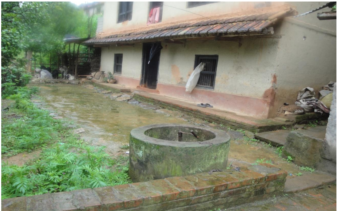
Figure 8. Biogas Plant without Toilet Attachment
