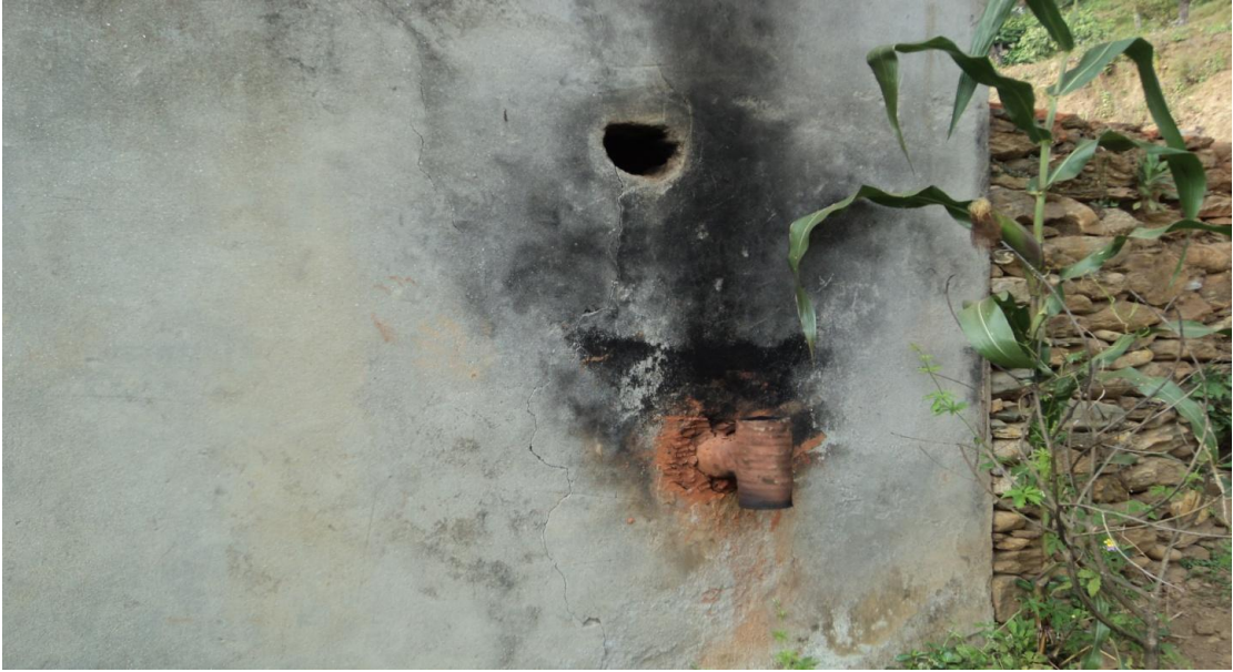
Figure 7. Chimney Outlet of Mud ICS
