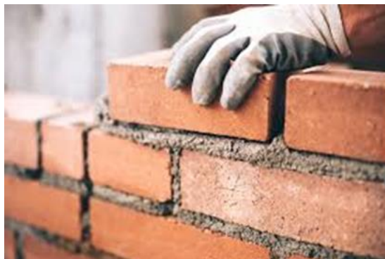
Fig.2. Construction of a wall
